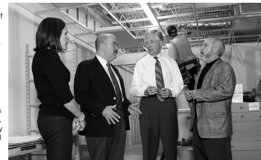
County Councilmember George Leventhal, (2nd from left) Saint Mark Presbyterian Church Pastor Roy Howard and member Barbara Welsh discuss construction progress with Dick Pavlin, Executive Director.
